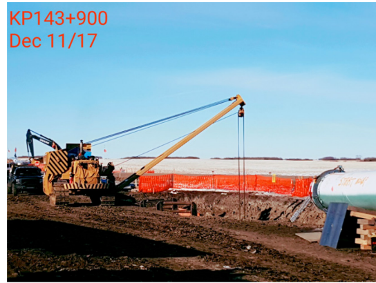
2. Track bore lower in – Km 143+900 – Dec 11, 2017
