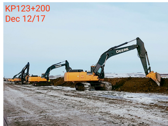
4. Backfill – Km 123+200 – Dec 12, 2017
