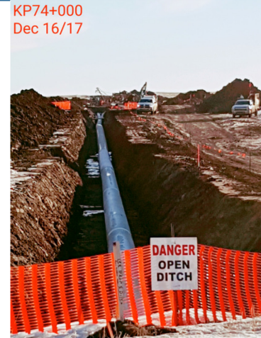
14. Backfill tie-in -74km+000 – Dec 16, 2017
