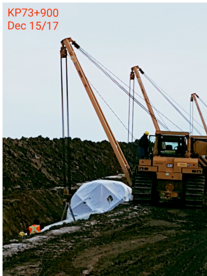
11. Tie-in - 73km+900 – Dec 15, 2017
