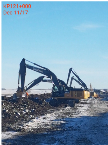
1. Backfilling – km 121+000 – Dec 11, 2017
