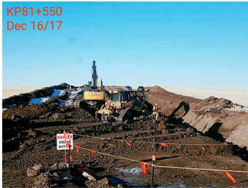
13. Backfilling tie in - 81km+550 – Dec 16, 2017
